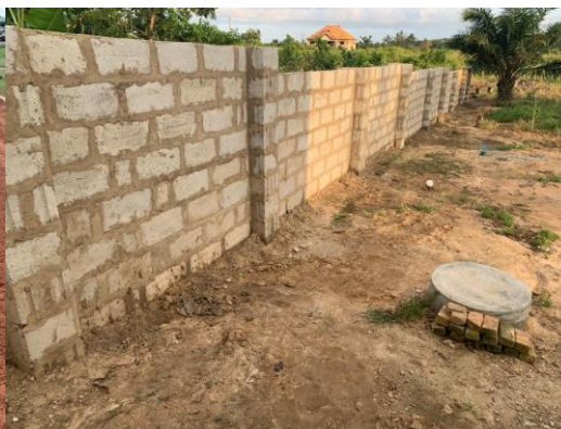
MTC wall in progress
